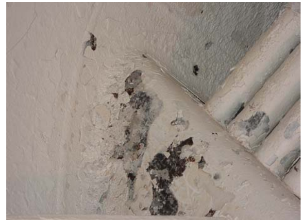
Scale in boiler side is soft and easy to clean
